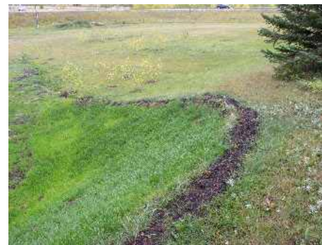
Installation of compost blanket over lockdown netting
