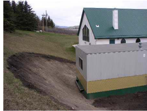
Installation of compost blanket over lockdown netting
