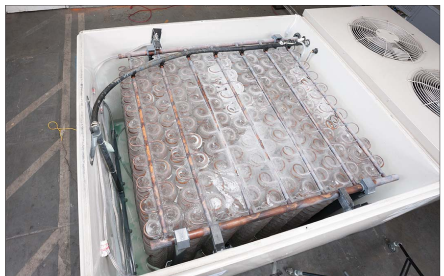
Ice Energy’s system freezes 450 gallons of water at night to offset daytime air-conditioning. Photo credit: Ice Energy
